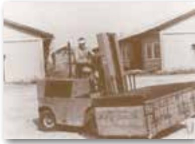
(Fig. 17) Vietnam 1973, arrival of equipment for component fabrication. Klaus Oschatz at work
